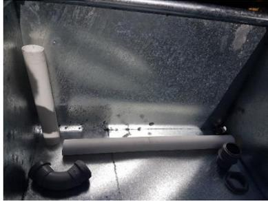
The overflow upstand (upright piece) should come up to 10cm below the lip of the planter when fitted to the bend (including the leaf guard). The base drainage pipe (horizontal piece) should fit the length of the planter including the bend (with some allowance so it can be fitted easily).
