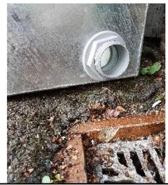
The planter should be located so it drains to the existing drain at the base of the downpipe
