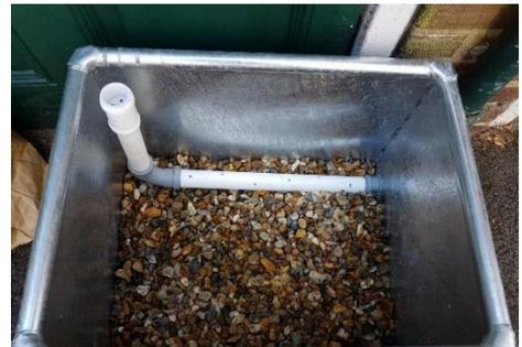
The gravel can be used to prop up one end of the base drainage pipe so it slopes slightly towards the outlet. Keep adding gravel until the pipe is just covered.
