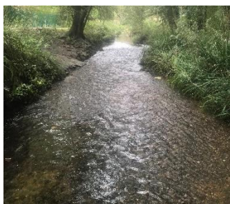
Ewell Storm Tanks (Photo thanks to Robb)
