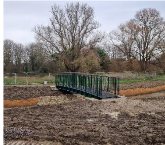
Chamber Mead bridge
